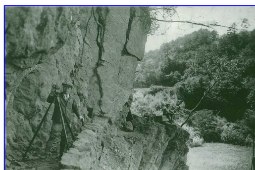
Photo 28: Surveying during mountainside irrigation canal construction
