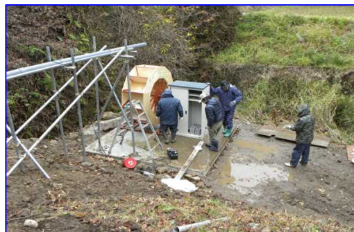
Photo 46: Research group setting up power generation equipment
